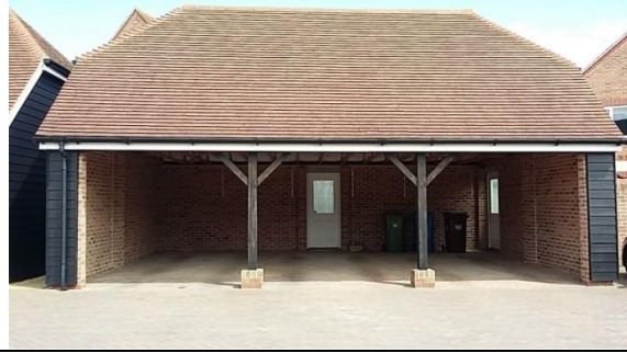
Figure A4 – An example of a parking barn in a communal parking courtyard.
